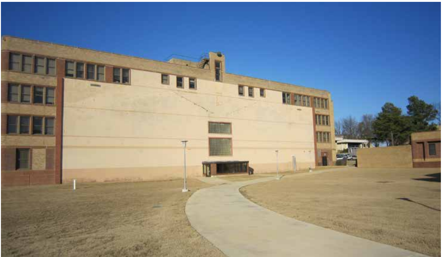
South facade of Business Building
