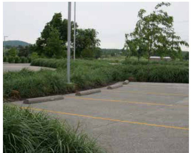
Pervious Concrete Paving
