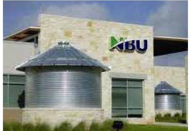
Above ground cisterns can be visually appealing and used as educational tools
