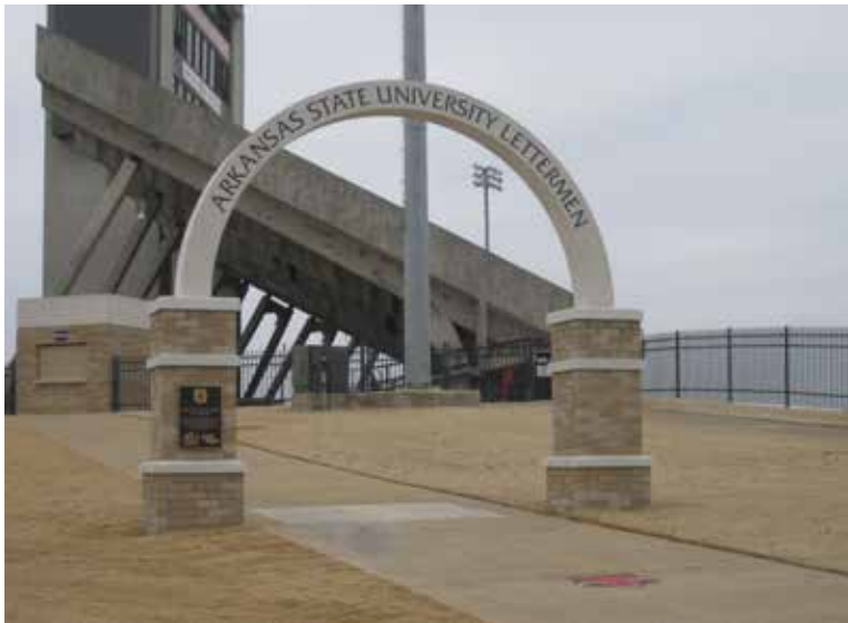
Southwest entry gate to Liberty Stadium
