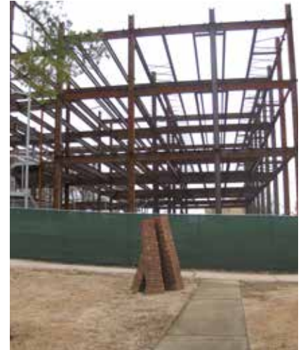
Existing Building Under Construction
