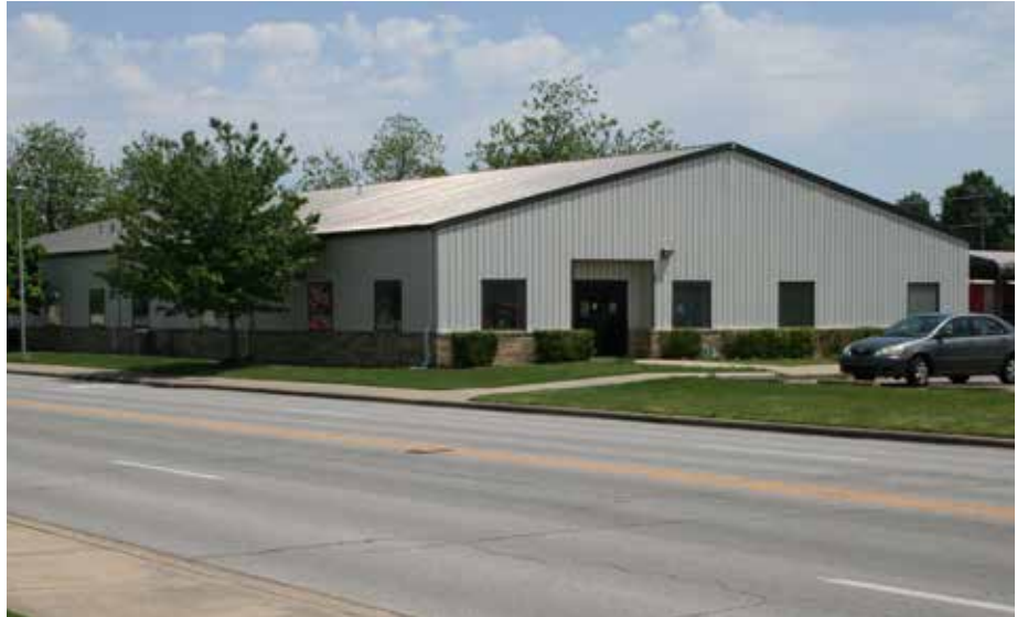
The existing Childhood Services building does not provide enough office and storage space.
