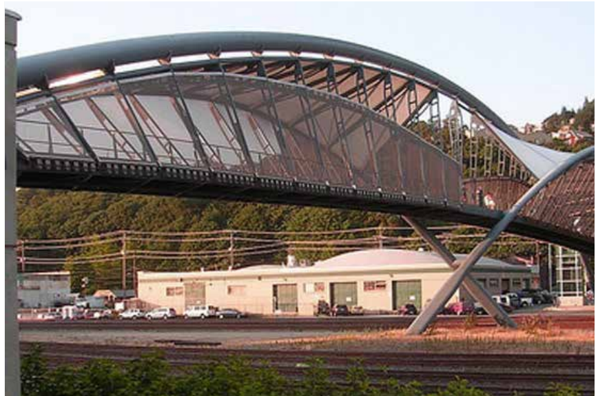
Pedestrian crossing over railroad tracks Elliot Avenue Helix Bridge, Seattle, WA
