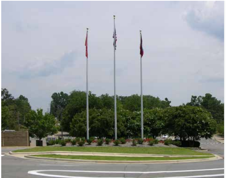
While the existing landscaped vehicle turnaround will no longer have a vehicle traffic role, it should be modified to become the Aggie Road Pedestrian Gateway.
