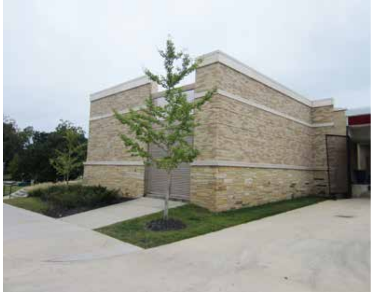
Appropriate Screening for Utilities
