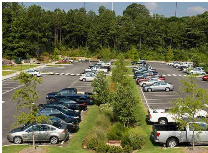
A bioretention area is located in the center of the parking lot to capture stormwater.
