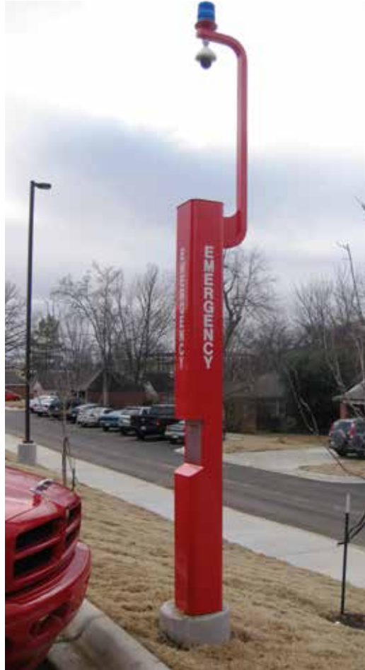
A new Talk A Phone emergency call box (without WEBS) on main campus.
