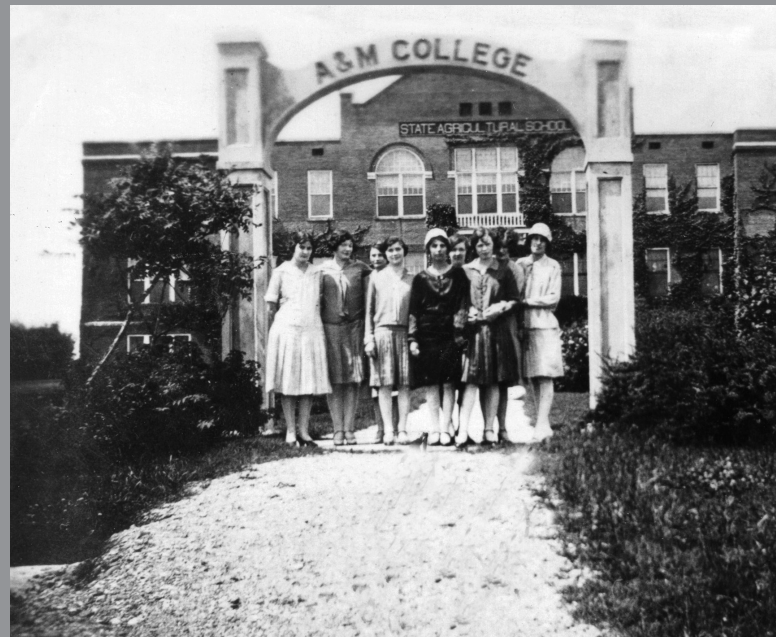
This photo includes the original Administration Building, which burned in 1931.
